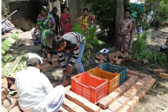
FLD on Use of zero energy cool chamber to maintain quality and extend post harvest life of vegetables
