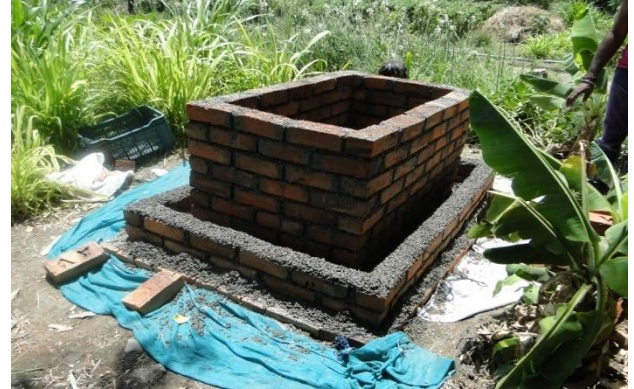
FLD on Use of zero energy cool chamber to maintain quality and extend post harvest life of vegetables
